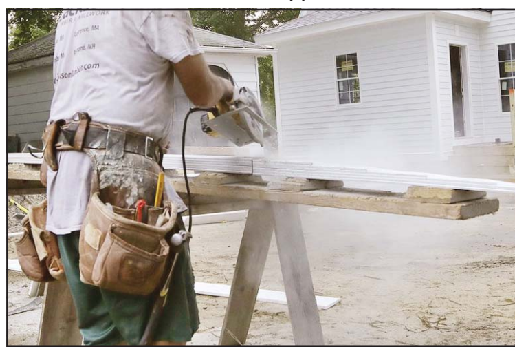
In this file photo, a carpenter works on a construction site in North Andover, Mass. On Friday, Jan 17, the Commerce Department reports on US home construction in December. (AP)
